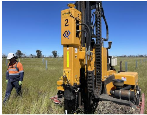
Photo 10: Piling rig on site.
